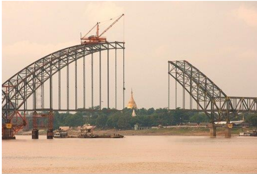
Bridge being constructed over the Irrawaddy River
