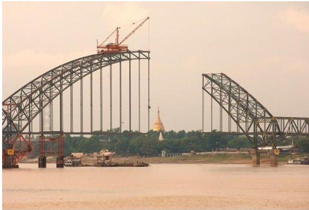
Bridge being constructed over the Irrawaddy River
